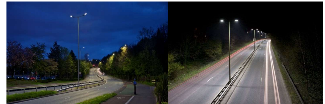
Figure 5—11 Precedent image for lighting of roads in the M3 and C2 category. Dense vegetation on both sides of the road blocks the light and shields the natural environment in the interior areas of the natural reserves
