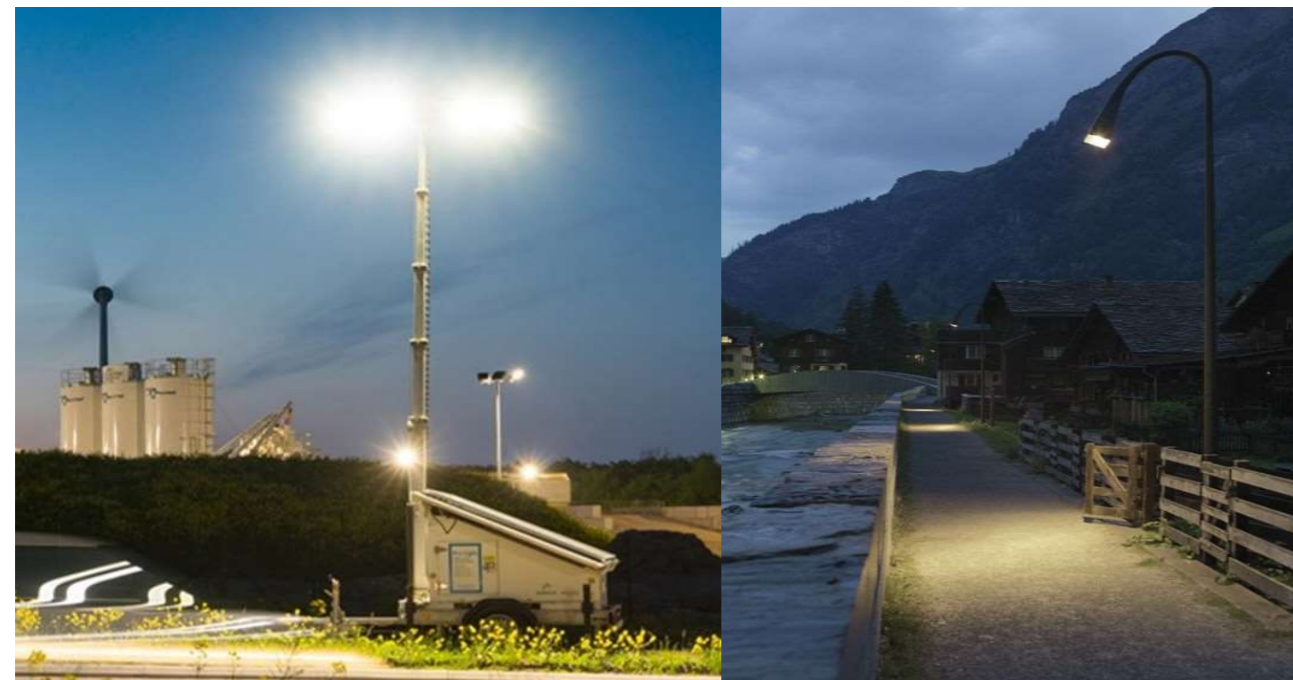
Figure 5—4 Comparison between high and low mounting scales. Image on the left shows large scale lighting column without any glare control and the image on the right shows a smaller column with controlled lighting distribution providing light to the path only
